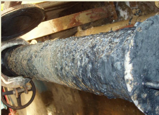
Figure 3. Slime inside shower bar rich of iron sulfide deposit— indication of anaerobic growth
